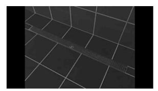
Close-up of a finished shower grate with the recommended 100mm from wall and 50mm from each side wall.
