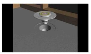
Recess concrete or AC sheet using a grinding wheel so that the puddle flange sits flat with the floor. Glue screw the puddle flange into position. Refer to manufacturers directions
