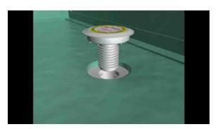
After the waterproofing is complete re-install puddle flange cap to prevent any building debris from entering plumbing untill ready to bed and tile
