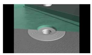
Have approved waterproofing contractor waterproof the area insuring the membrane goes onto and into the puddle flange
